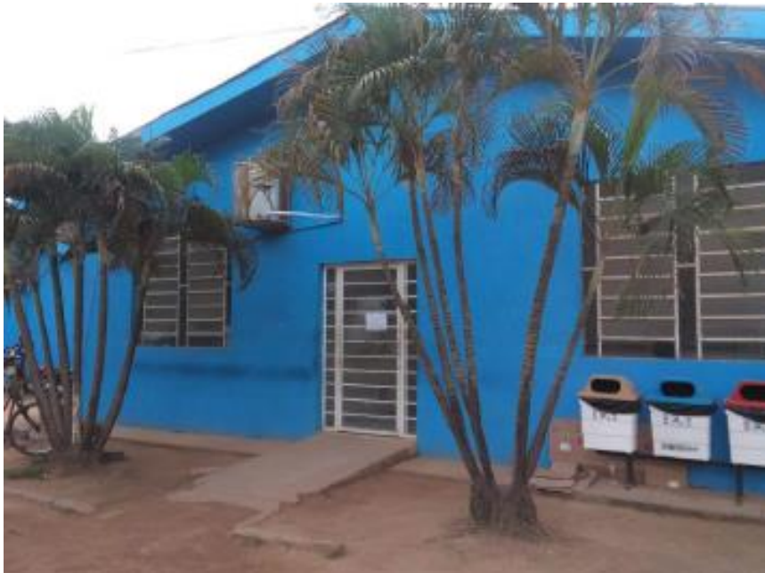
Figure 11 - Cujubim Hospital that benefited from donations of materials for its renovation.
