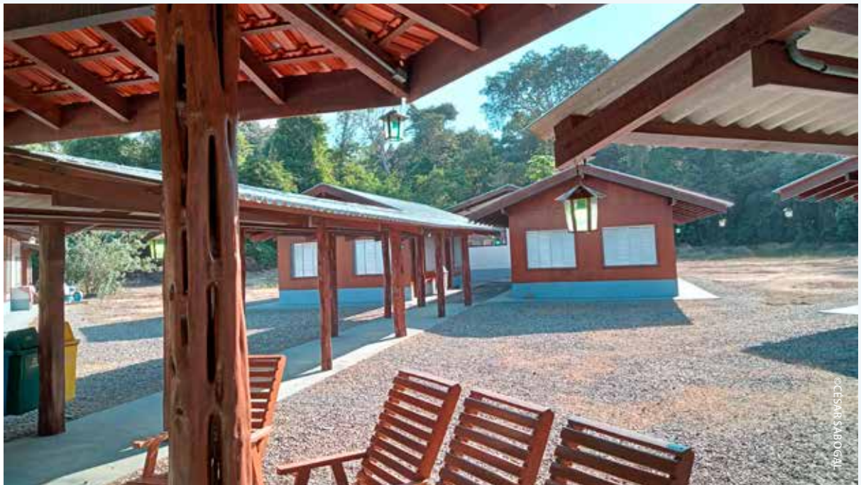
Dormitories for employees at a permanent forest camp
